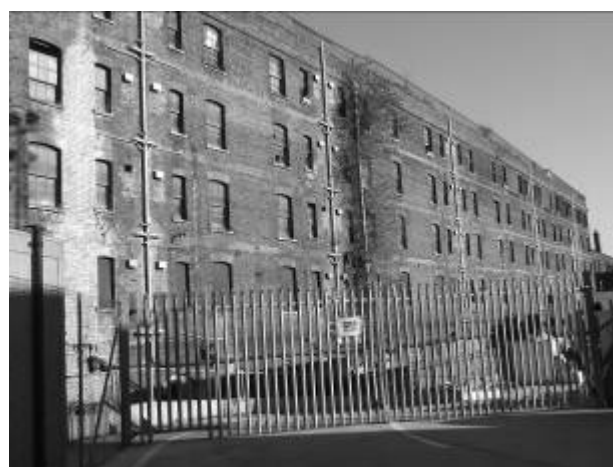
The Culross building 1891-2, facing the bulldozer
